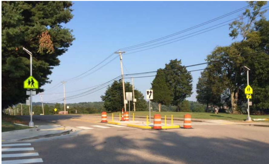
Pedestrian refuge island on George Williams Road
